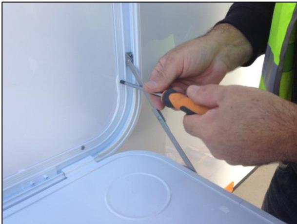
Please note that the silicone/sealant is not only for waterproofing the installation holes. It will also add strength. In most cases you will not screw the picnic table frame into a wall stud, therefore it is vital to use adequate, appropriate silicone/sealant.
