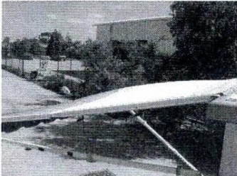
SHOWS CURVED ROOF RAFTER IN POSITION
